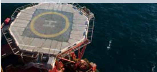
Helideck Monitoring System
